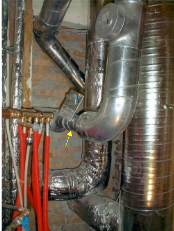
Figure 2.7. The calibrated orifice.
