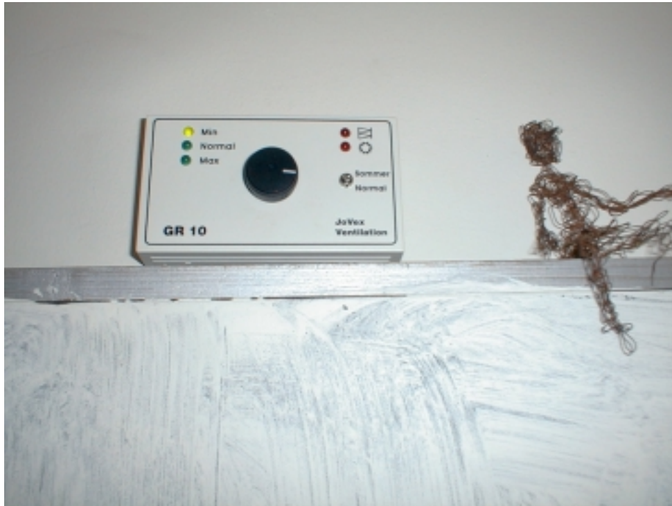
Figure 1.14. The control panel from which the occupants of the dwellings may control their ventilation systems.
