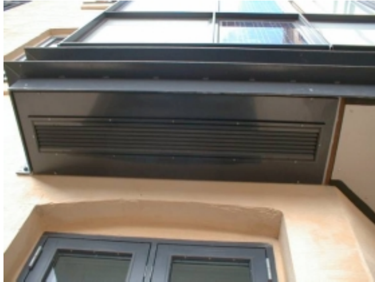
Figure 1.5. The inlet to one of the solar walls.
