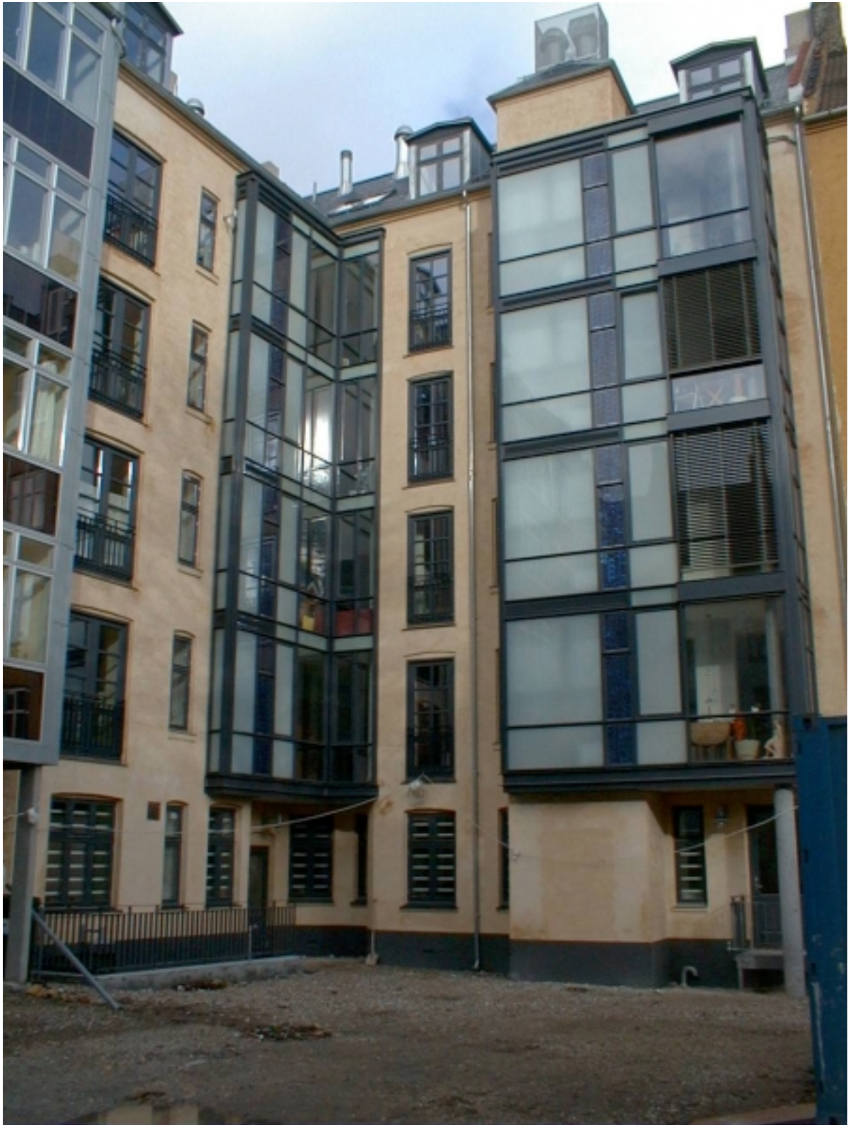
Figure 1.3. The facades facing the courtyard after renovation.
