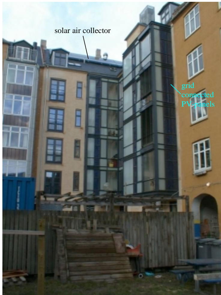
Figure 1.13. The grid connected PV-panels on the south gable of the solar wall on Sundevedsgade 14 and the solar air collector array on the roof of Tøndergade 1.
