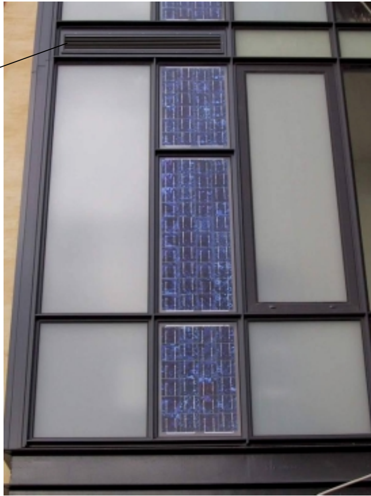
Figure 1.12. Close up of the PV-panels for one dwelling.
