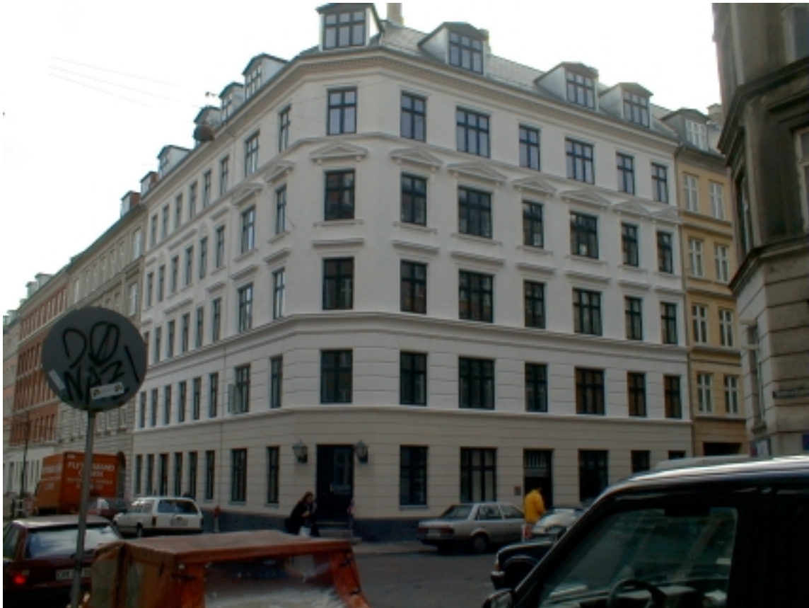
Figure 1.2. The facades of the building after the renovation.
