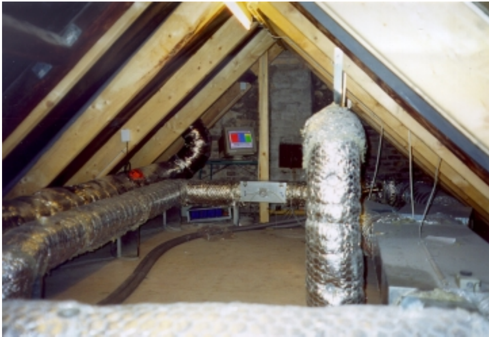
Figure 2.10. The attic at Tøndergade 1 with the PC/data logger system located at the back wall.
